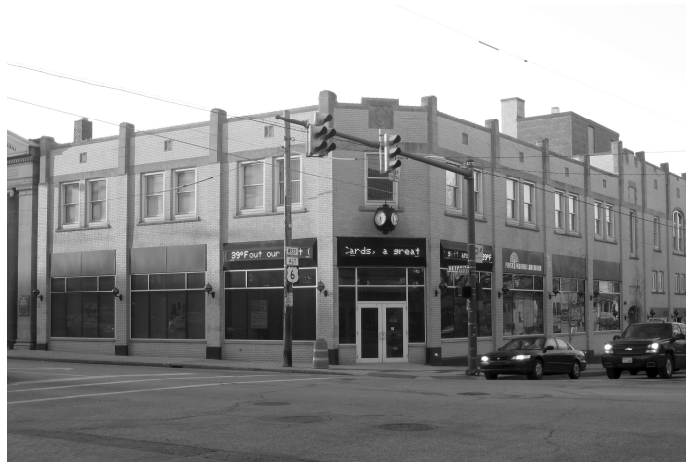
14800-06 Detroit Avenue 2012. The same basic building after numerous modifications still stands there today.
